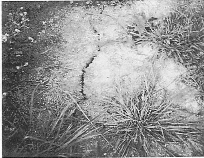
Photograph showing the cracks in the burn area (taken August, 1984).
